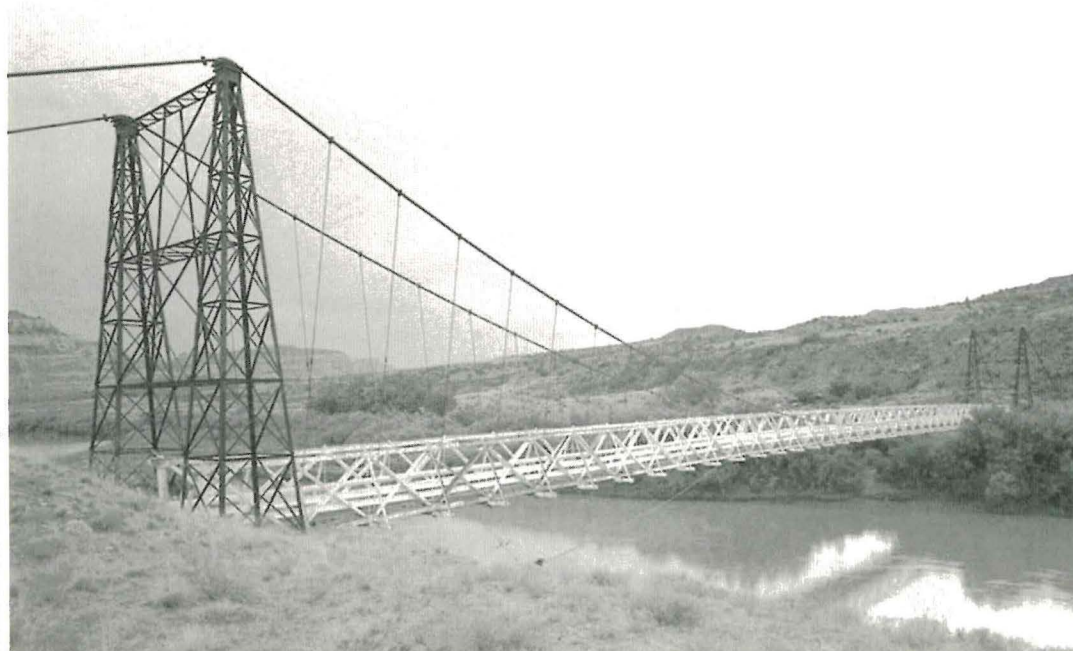
Dewey Bridge, Moab, Utah.
