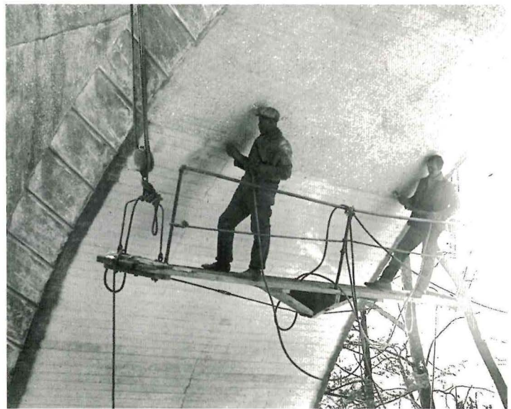
Workers finishing the intrados of the arch.
