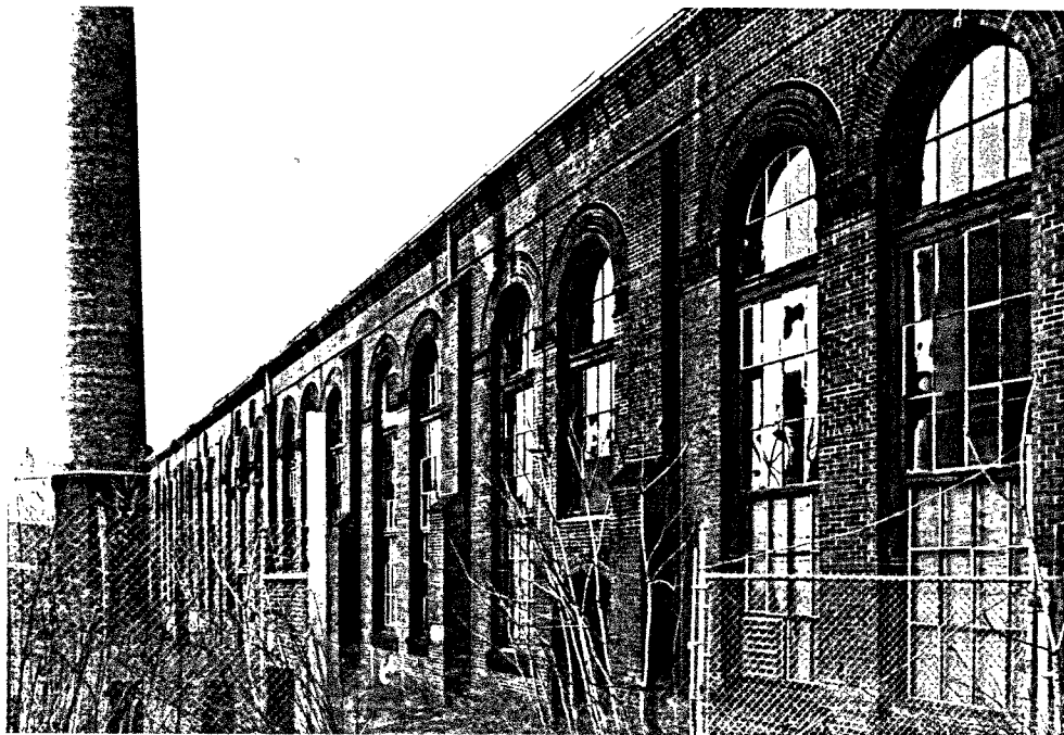
COAL STREET STATION
