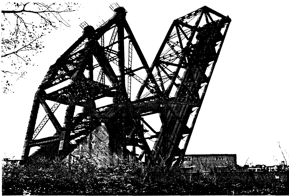
PATERSON-NEWARK BRANCH ERIE RR Abandoned bascule
