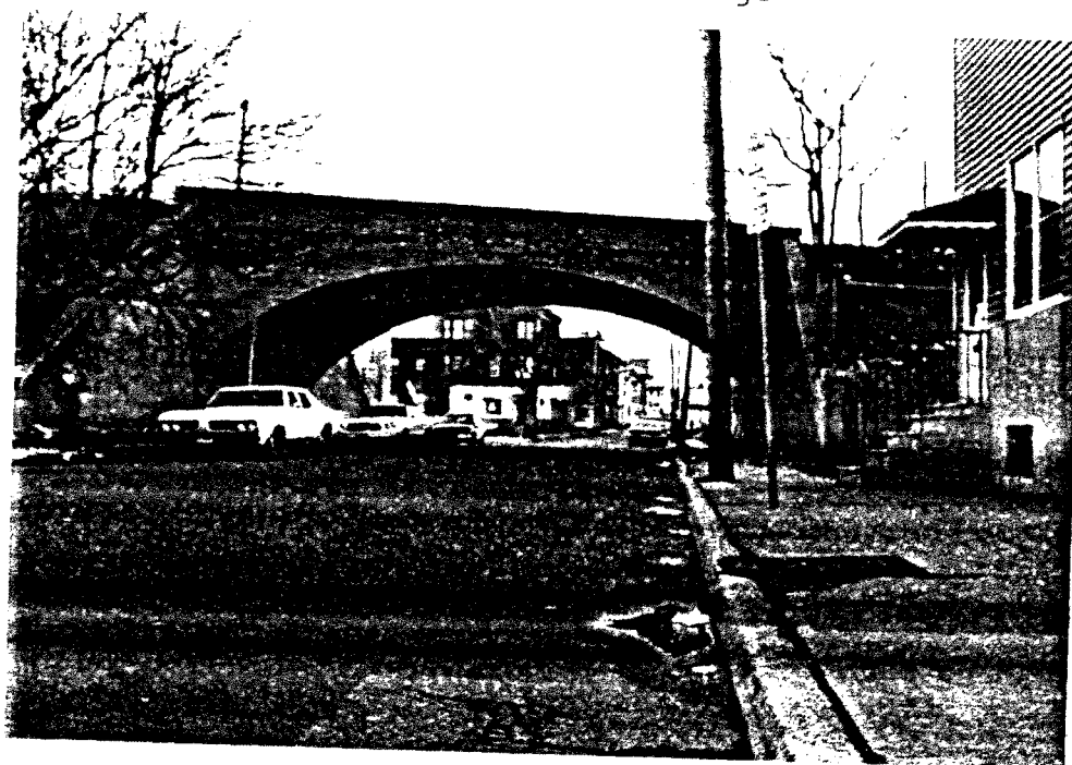
Jackson Street Bridge
