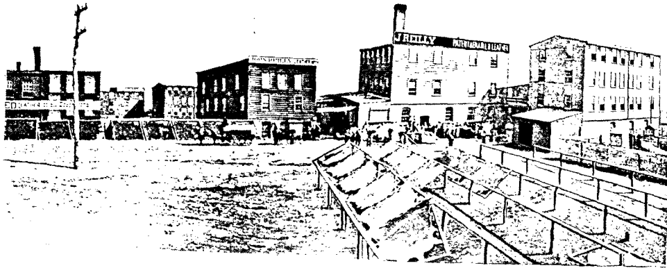
JOHN REILLY CO. Newark, NJ Illustrated, 1893, p. 92. extant building is at far left
