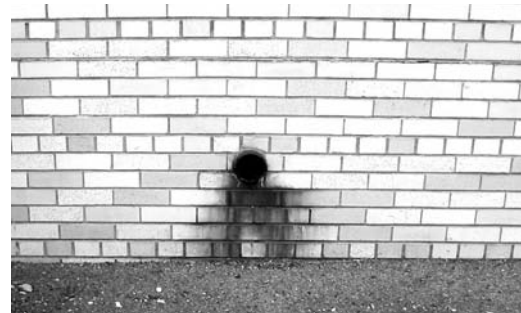
Floor drain outfall corresponding to sectional drawing.
