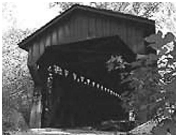
Salem-Shotwell Covered Bridge.
