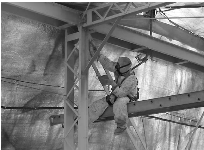
Inside the cocooned bridge, workers removed lead-based paint and applied new paint.
