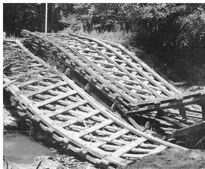
The collapsed Town-lattice trusses of the Salem-Shotwell Bridge, June 2005. The trusses have since been salvaged and will be repaired and re-erected at a new location.
