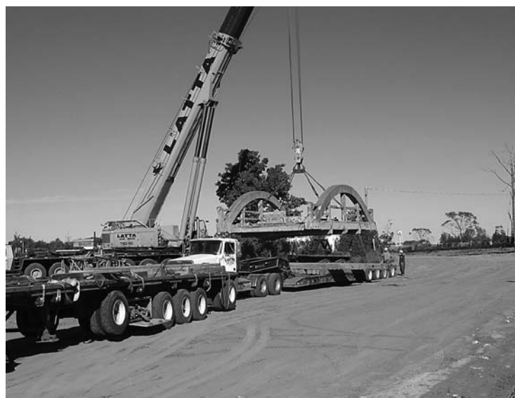
Lifting the bridge off the flatbed truck at the Wellington County Museum, Oct. 2004.
