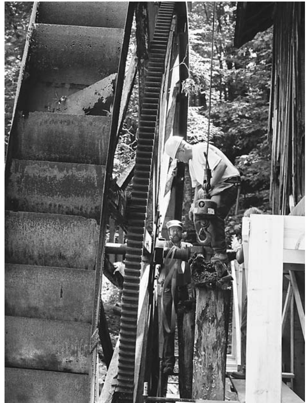
Lou Mogavero of Dearborn, MI (front) and Will Hines of Greeneville, TN, prepare for the crane to lift the waterwheel just enough to slip a temporary support in place.
