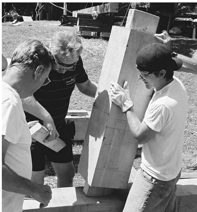
Jerry Donahoe of Clearwater, FL, Jeffrey Finch, the technical expert, and Patrick Willis, of Canton, NC, check the fit of the beam that will support the millstone shaft support beam.
