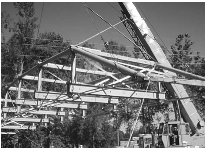
A crane prepares to set the restored Aldrich Change Bridge on its new abutments.
