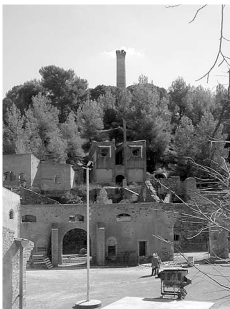
The remains of the smelter at the Bellmont lead mine.
