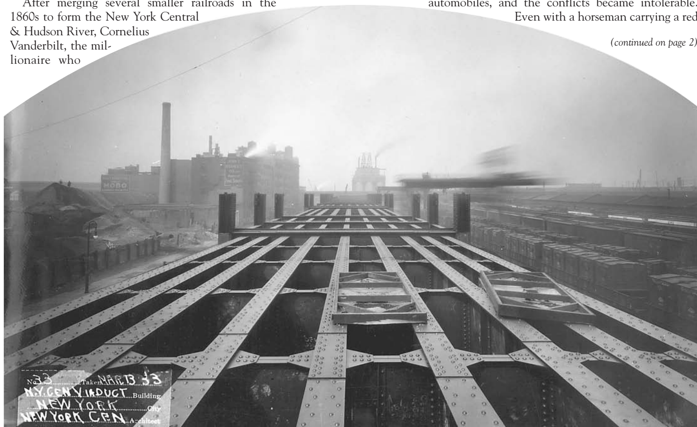
The High Line's very heavy construction is in evidence before the reinforced concrete deck is laid down. March 13, 1933.
