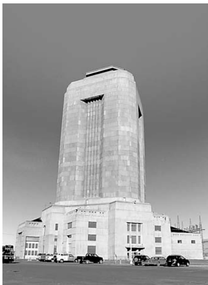
In addition to power generation equipment, the Fort Peck Dam Powerhouses also contain the 15-story surge tanks that assist with controlling the water flowing through the facility.
