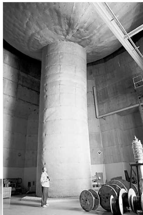
A Fall Tour participant marvels at the base of a 4.5-million-gallon surge tank at the Fort Peck Dam.
