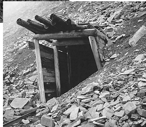
Shaft for waste rock from the Hiorthamna Mine.
