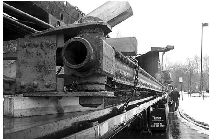
Doty Road Bridge’s Phoenix Column upper chord aboard a flat bed trailer on its way back home to Phoenixville, PA.
