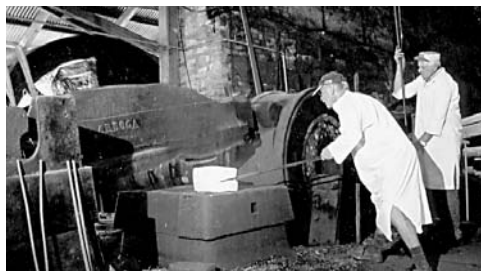
Working the Lancashire forge at Karmansbo: The heated iron is lifted from the hearth onto a small cart (left), transferred to the “mumblingshammer” (middle), then to the rolling mill (right).
