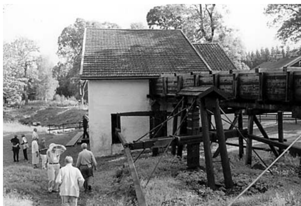
Magnificently reconstructed, the waterwheel at Pershyttan drives the stångång (left), which once transmitted power for pumping to nearby mines by means of reciprocating rods.
