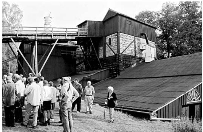
The blast furnace at Engelsbergbruk, built in 1779 and rebuilt in 1878, is one of the few earth-and-timber furnaces preserved in Sweden.
