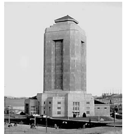
Powerhouse at the Fort Peck Dam, showing the housing for the giant surge tank.
