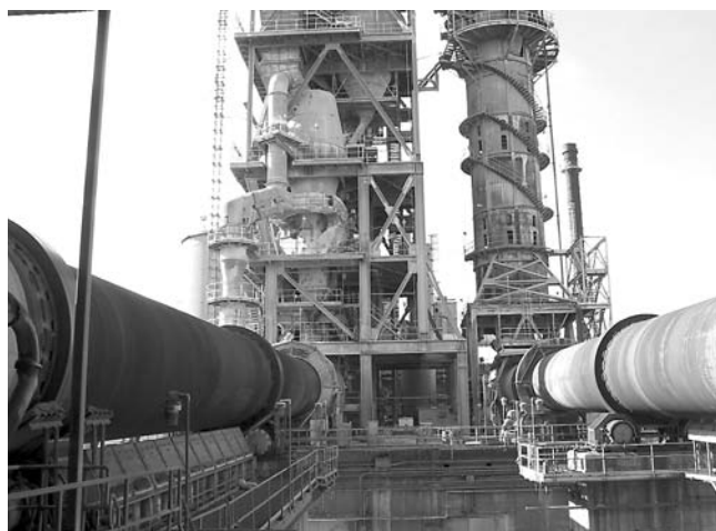
Rotary kilns, Hercules Cement.
