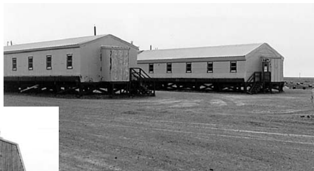
ARMCO's—prefabricated metal buildings on timber foundations—provided the primary shelter for soldiers and workers at FOX-M.
