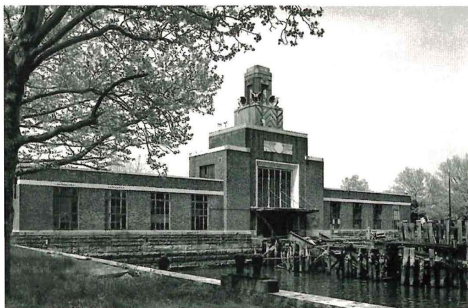
Ellis Island Ferry Terminal, prior to restoration.
