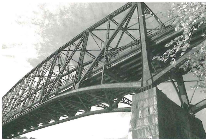
Schell Memorial Bridge.
