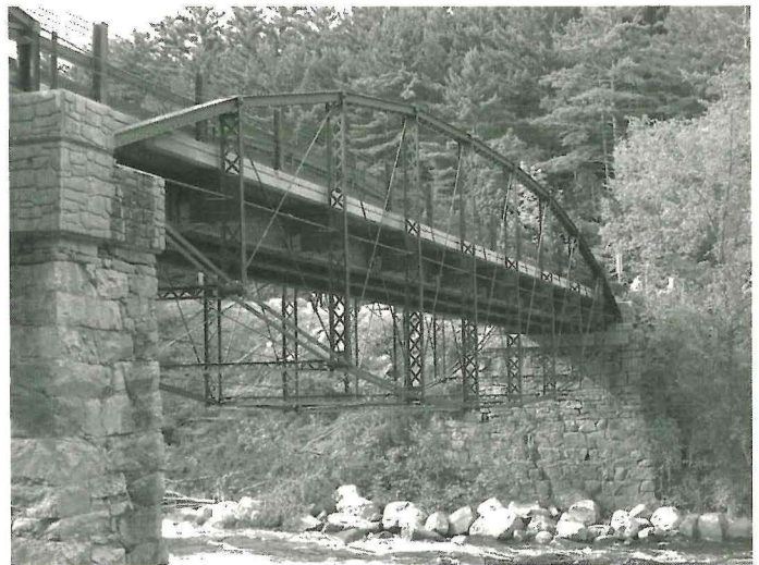
The Hadley Bow Bridge in 2006, following completion of the project that resulted in a new steel superstructure with the 1885 trusses attached to the exterior floorbeams.
