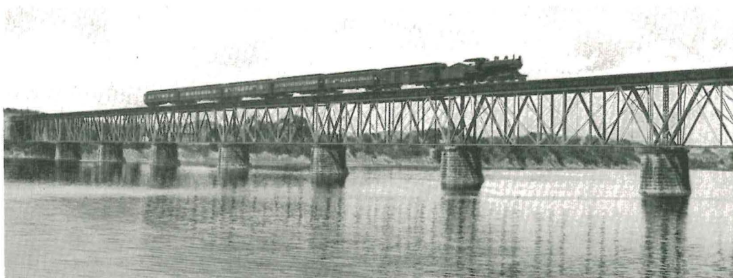
Photograph, circa 1902, of the 1894 bridge with Whipple trusses supplemented by the insertion of Warren trusses.
