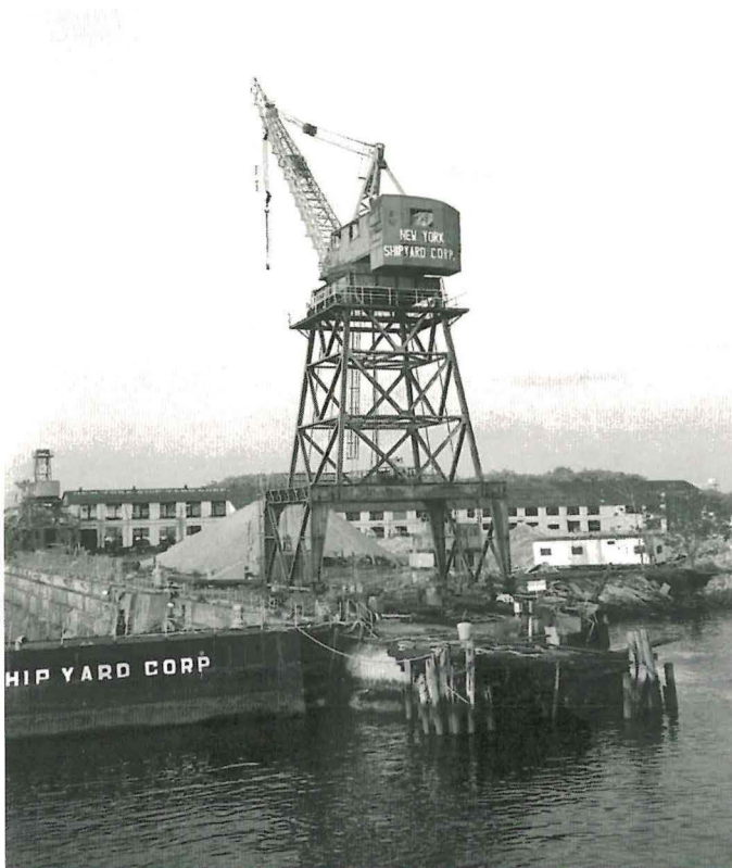
One of the remaining gantry cranes, which IKEA plans to use as part of a maritime promenade. The large pile that looks like gravel is ground-up building debris. The estimated 15 truckloads of debris mysteriously disappeared from the site over MLK weekend in January. The NYPD is investigating.
