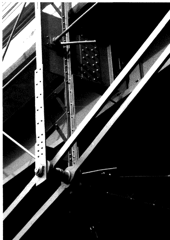
Detail showing the connection of the stub of the original floorbeam to a new steel beam that now supports traffic loads.
