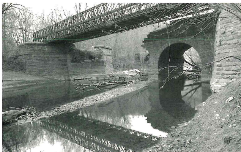
The remaining stone arch and abutments of the Catoctin Creek Aqueduct. The center span collapsed in 1973 to be replaced by the Bailey truss bridge.
