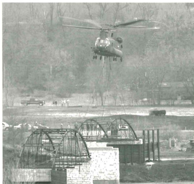
A Chinook helicopter places the Hale Bridge's center span on its new stone-faced concrete piers in Wapsipinnicon State Park.
