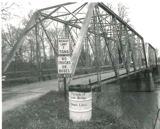
Lost Bridge in Miami County, IN, built in 1915, has served as the inspiration for a county-wide "save our bridges" movement.
