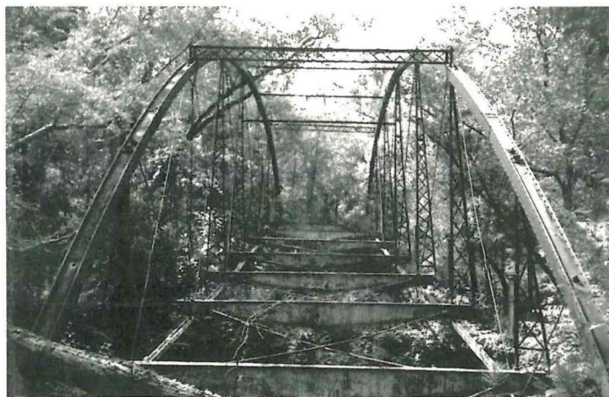
Black Warrior Bridge as it currently appears abandoned in the woods of northern Tuscaloosa County. It will be relocated to a trail atop the levy in Northport, near its original location over the Black Warrior River.
