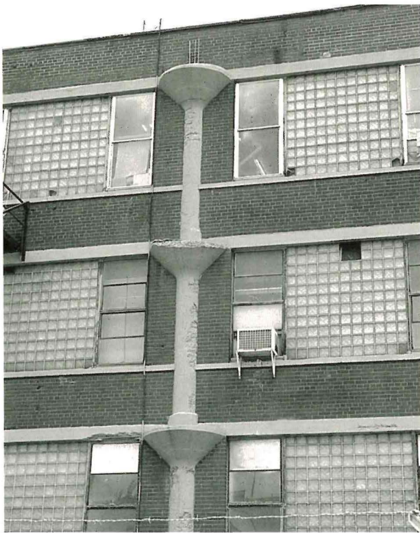
The reinforced-concrete mushroom-column construction of this former RCA Victor factory, built about 1920, is clearly expressed. It now houses the Musée des ondes Émile Berliner that pays tribute to the inventor of the flat recording disk through an impressive collection of phonographs, radio receivers, tape recorders, and television sets. The museum held tours for several SIA groups.
