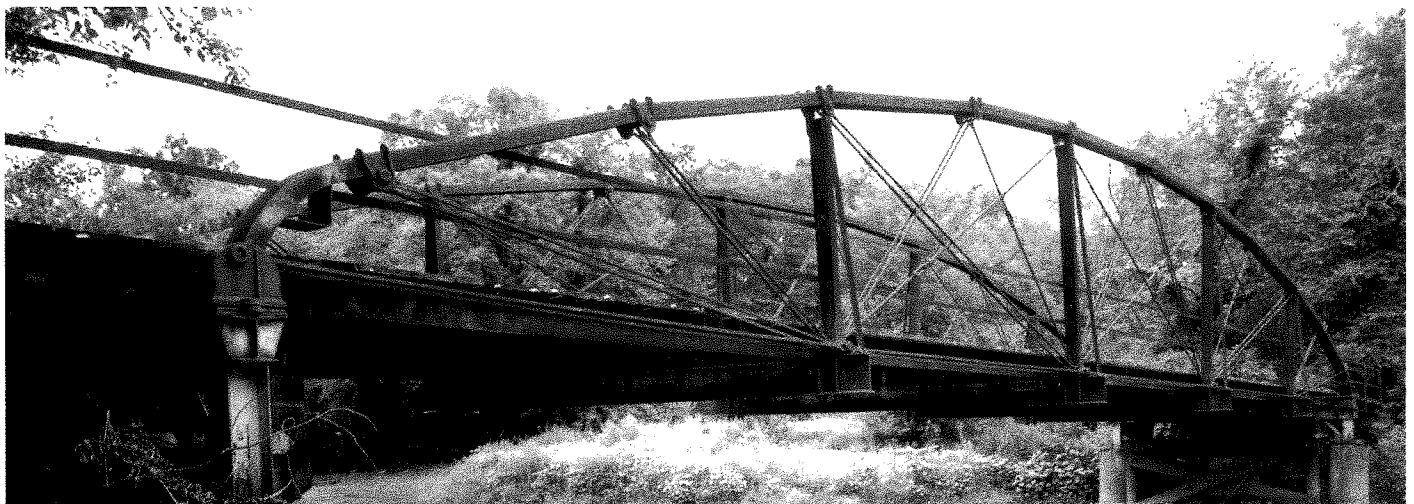
Figure 5: One of five extant Horton bowstring trusses in the VanLoon Wildlife Area north of Lacrosse, WI. Source: HAER WI-22B-2.
