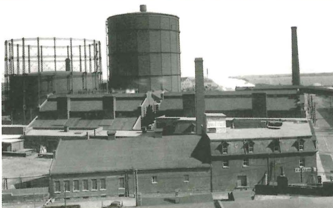
The Consumers' Gas Company water gas purifying buildings (1926) in front of two large gas holders. The short rectangular ventilation shafts identify the building. Source: City of Toronto, Consumers' Gas photographic collection, SC 34 - #340.
