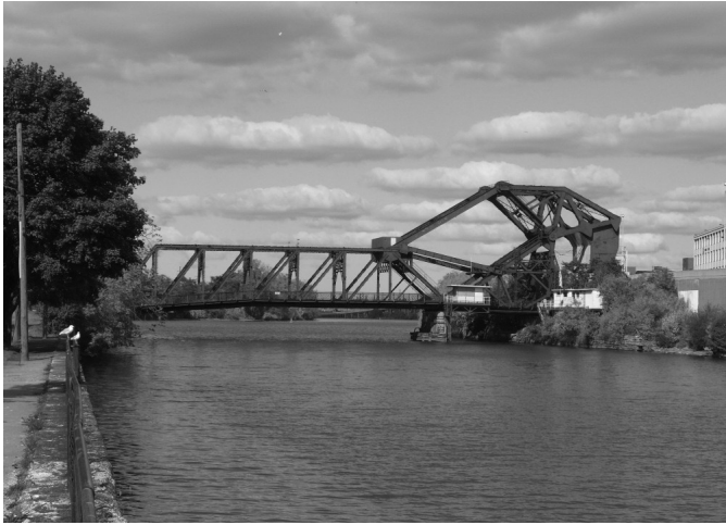
WEST FERRY STREET BRIDGE 1 West Ferry Street Buffalo
