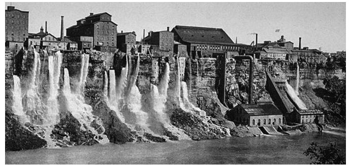
SCHOELLKOPF POWER STATION Niagara Falls State Park Niagara Falls, NY
