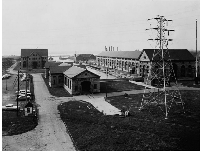
ADAMS POWER PLANT (POWERHOUSE NO. 1) 1501 Buffalo Ave Niagara Falls
