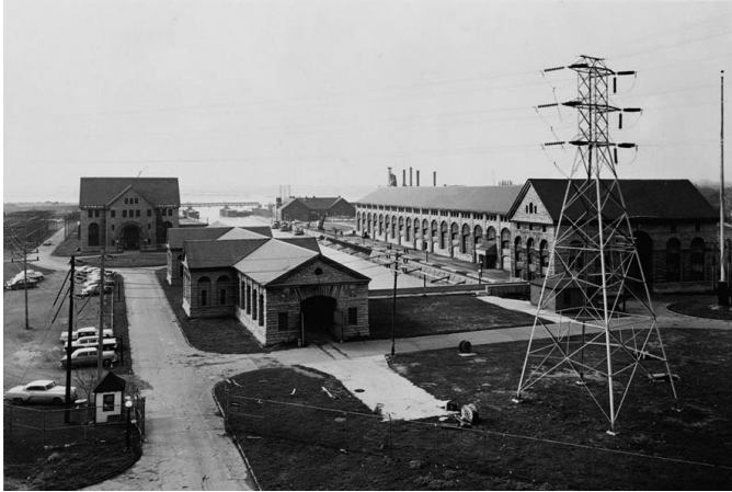
ADAMS POWER PLANT (POWERHOUSE NO. 1) 1501 Buffalo Ave Niagara Falls
