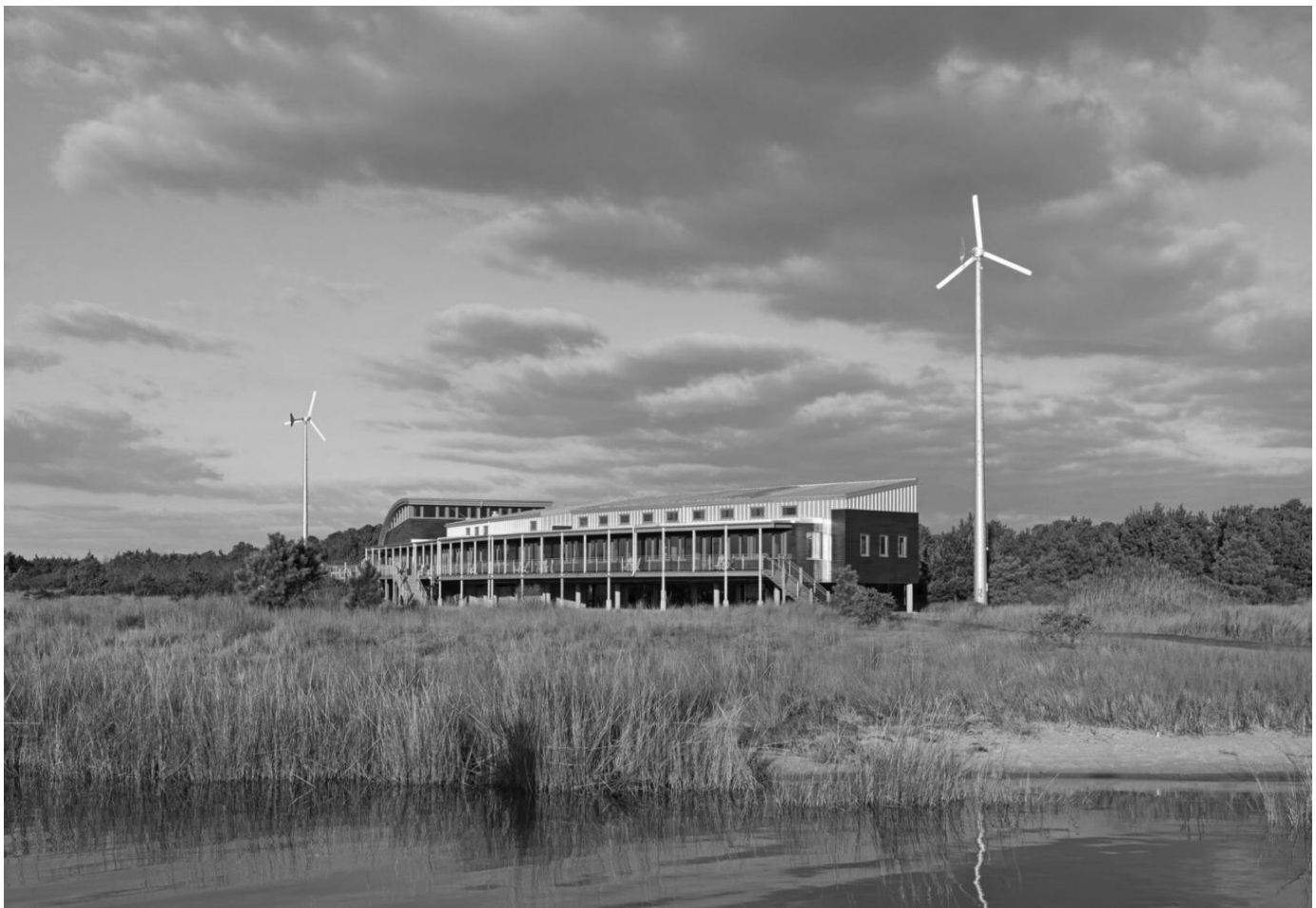
10-kW wind turbines flank the Brock Environmental Center helping CBF achieve net-zero energy consumption. Courtesy CBF.
