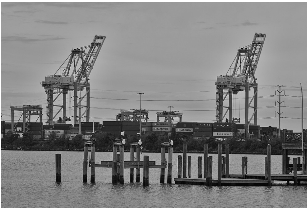
Container shipyard and cranes in the busy port of Norfolk. Carol M. Highsmith, 2019.
