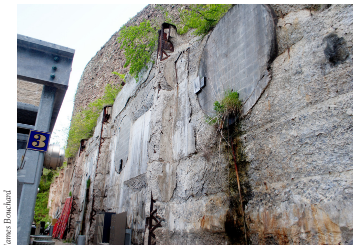
Penstock among the ruins of the Schoellkopf Power Station site.
