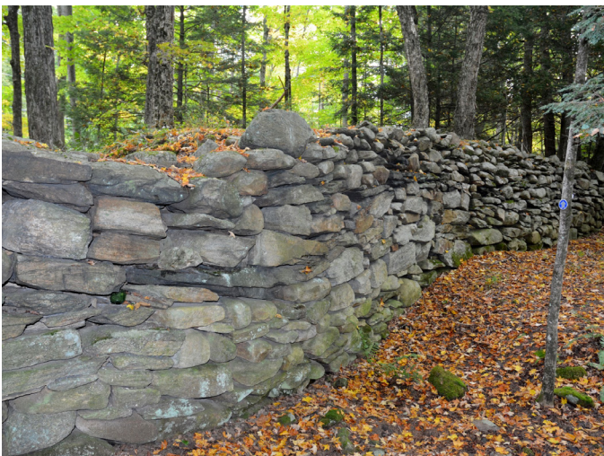
Graves Ironworks, handlaid 500-ft.-long stone berm along the canal feeding the ironworks, Sept. 2024.
