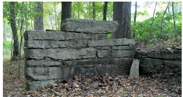
Graves Ironworks, section of cut-stone foundation of an ironworks building, possibly from a later period than the original dry-laid stone dam upstream, Sept. 2024.
