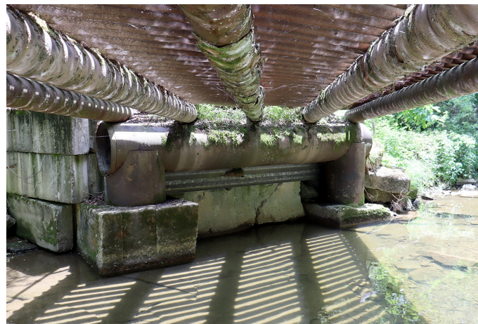
Underside of the bridge, showing the pipe stringers and the abutment constructed of pipes encased in concrete.
