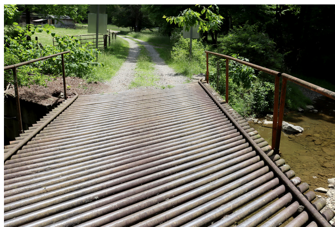
The 56 pipes comprising the bridge deck, aligned on the bridge skew.
