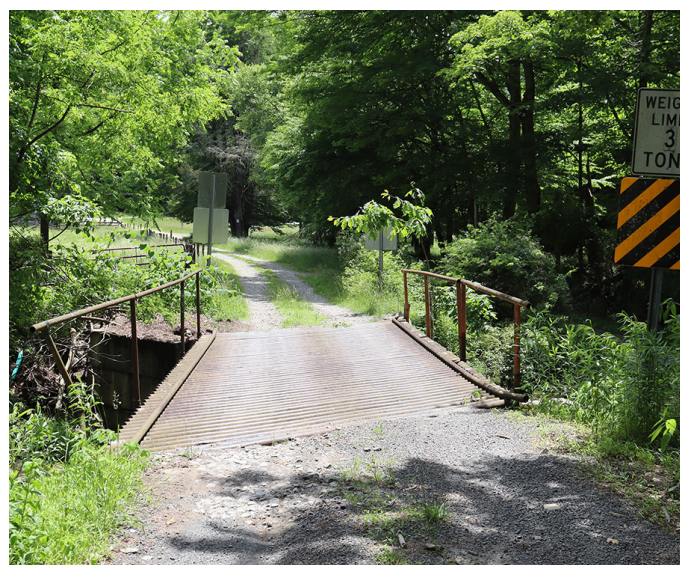
Deck view of the pipe bridge and unpaved Bucklick Road.
