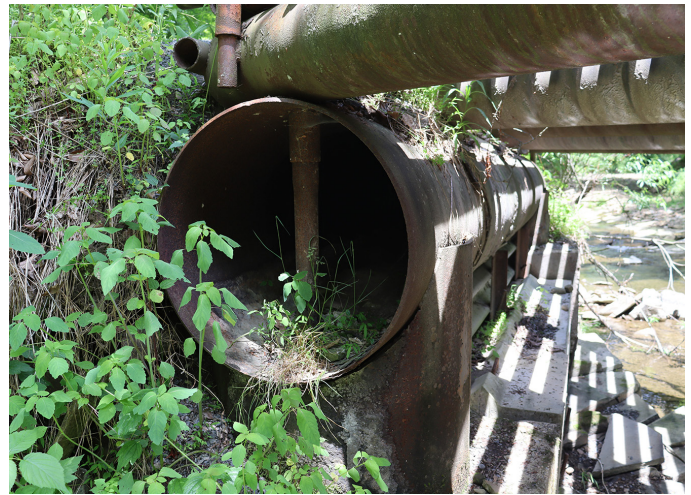
Side view of the abutment with the large pipe cap supporting the pipe stringers.
