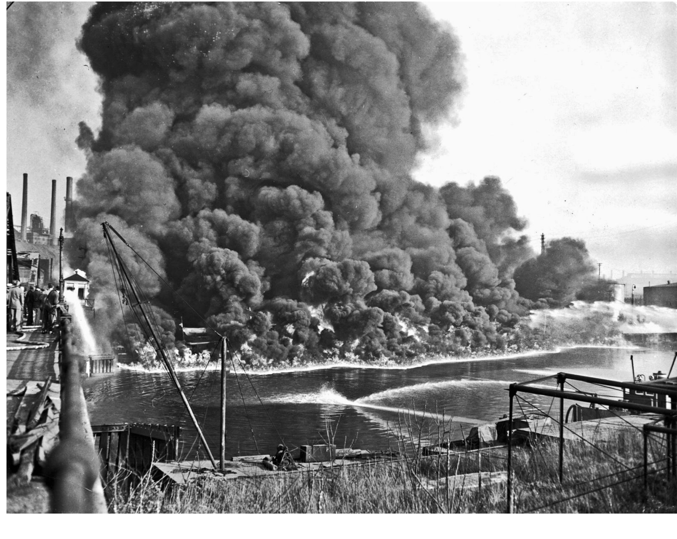
Buildings Also Damaged in $1,500,000 Blaze; Bridge Put Out of Order Fire that started on the oil-laden surface of the Cuyahoga River swept through the shipyard of the Great Lakes Towing Co. at 201 Jefferson Avenue S. W. yesterday afternoon, disabled the Jefferson Avenue Bridge and caused damage estimated nationally at $500,000 to $1,500,000.
