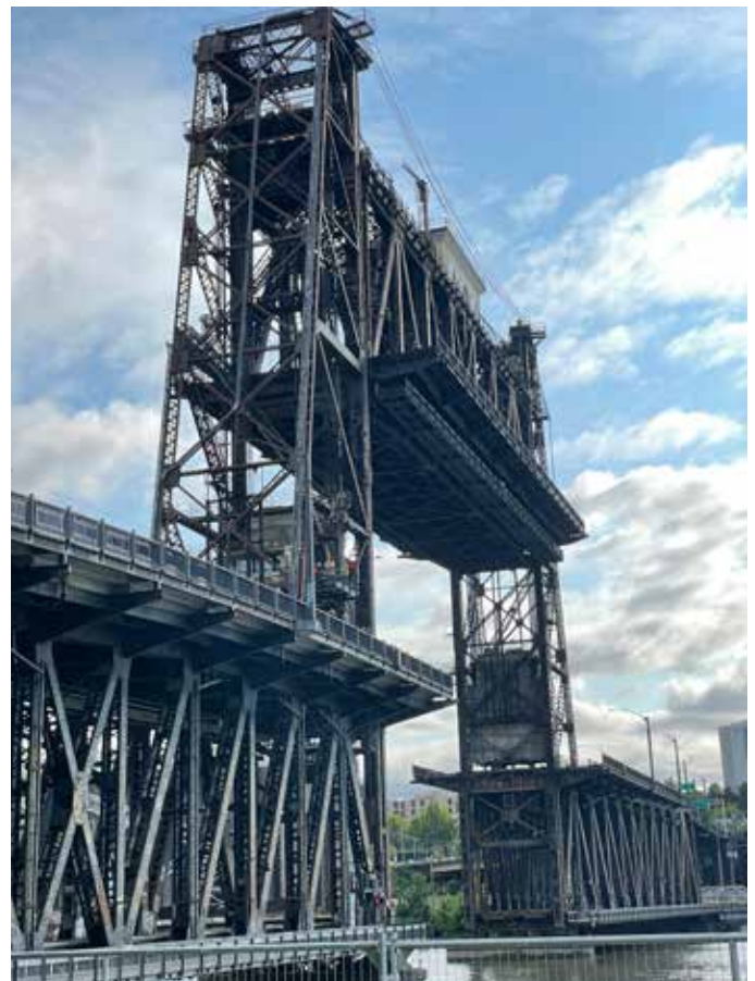
Both decks lifted on the 1912 Steel Bridge.
