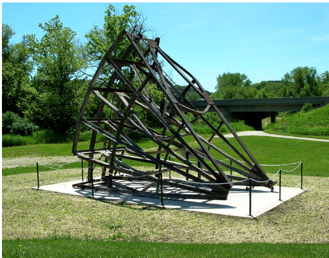
Remains of the last Tainter dam gate from the Lower Dam on the Upper Iowa River, displayed at Trout Run Park, Decorah, Iowa.
