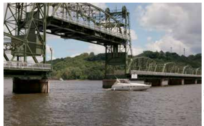
The newly rehabbed 1931 Stillwater Lift Bridge crossing the St. Croix River between Minnesota and Wisconsin, now converted to a pedestrian and bicycle trail bridge. Here restored to its original green paint.
