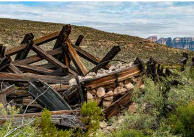
Middle of the terminal ruins looking southeast towards Mexico. Rocks in the crib are likely ballast and not ore.
