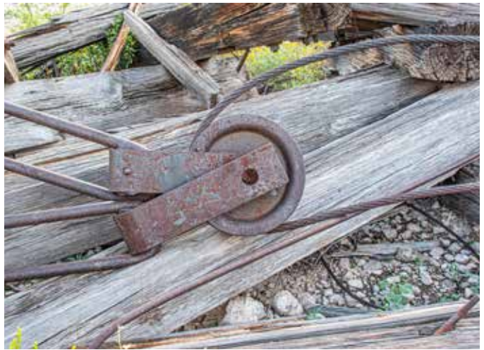
Pulley of uncertain function located in the tower remains seen in the first photo. One possibility is maintaining tension on the static cable.
