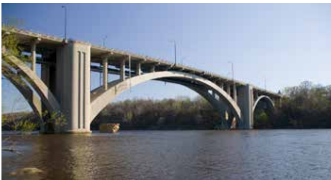
Named for Frederick William Cappelen, its Norwegian-American engineer who died during construction, the Cappelen Memorial Bridge's 400-ft. main span was the longest concrete arch in the world when it was completed in 1923. Crossing the Mississippi in Minneapolis, the bridge is shown here prior to its recent rehab.
