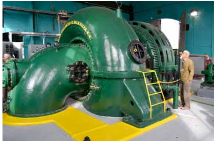
Verdi Hydroelectric Plant, turbine and alternator.
