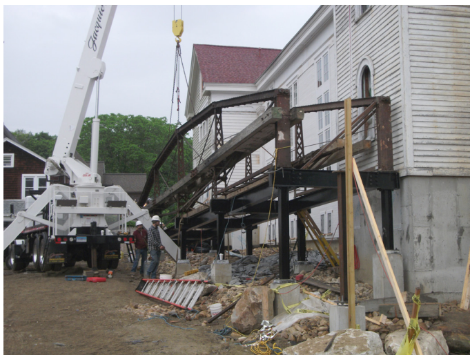
Installation of Great Barrington's 1888 Berlin lenticular-truss bridge at its new location.
