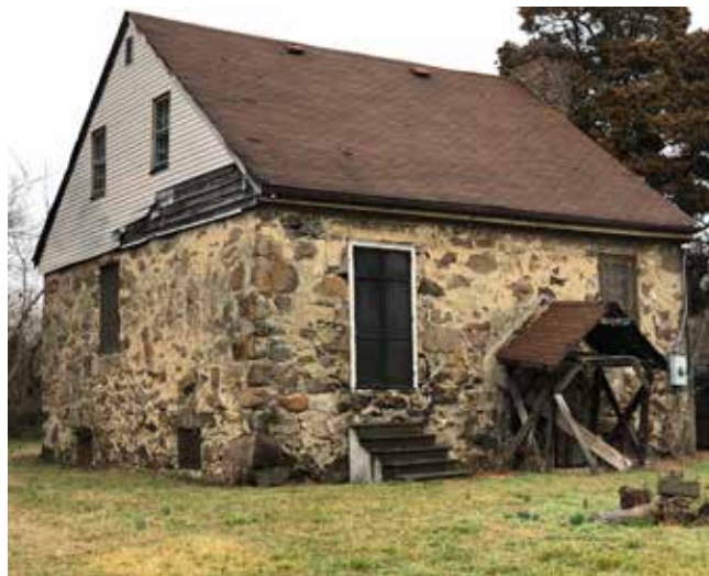
Canal keeper house on the Appomattox Canal, Petersburg.
