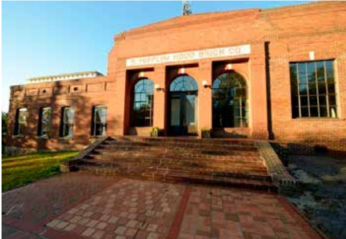
Main entry of the B. Mifflin Hood Brick Co. building.
