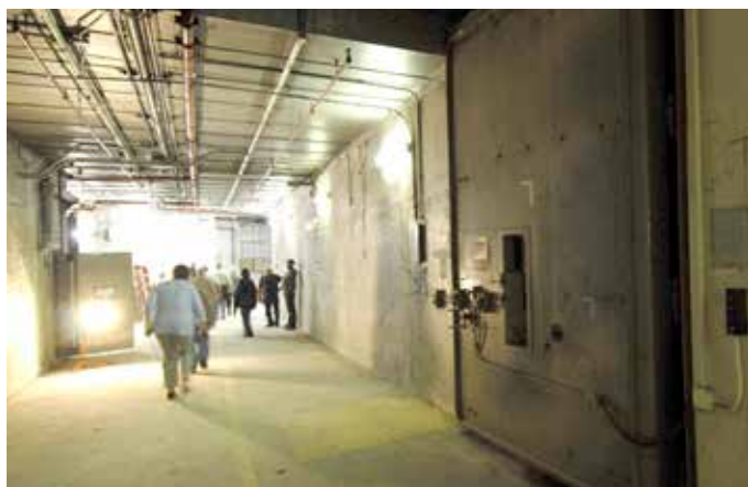
A blast door in the entry tunnel of T Building, Mound Laboratory.
