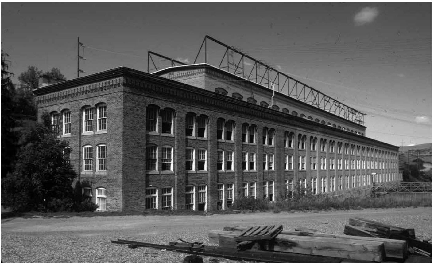
Rainbow Powerhouse, built just below Rainbow Falls in 1910, supplied electrical power to the copper mines at Butte and to the Anaconda smelter.
