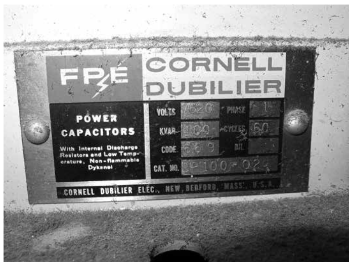
Manufacturer's plate on a Cornell Dubilier Electric Corp. capacitor. Note "non-flammable Dykanol." Philadelphia, Pa., 2014.
