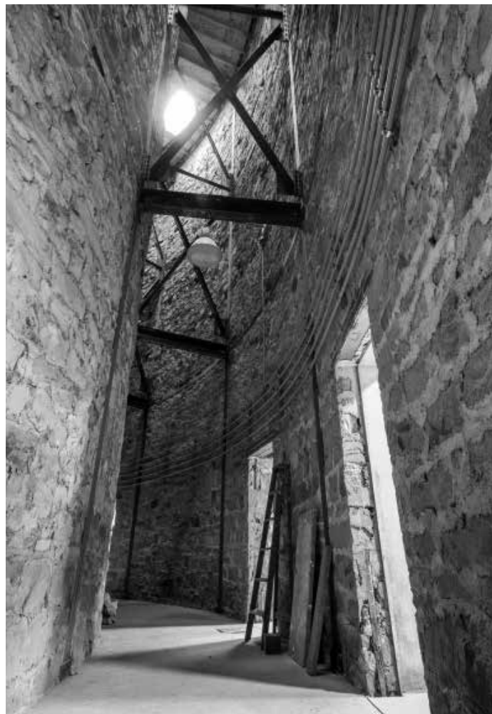
Interior stonework and steel frame of bandshell.
