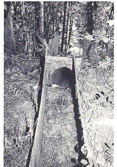
From the ditch, water was collected into a wooden headgate.
