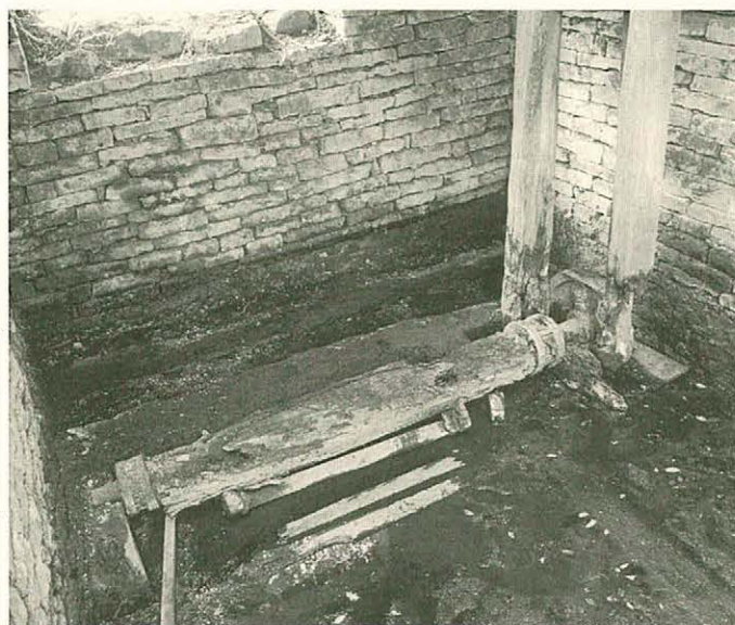
ABOVE: The flutter wheel remnants in the pit of the Staley sawmill are a rare surviving example of a once common water-power technology.
