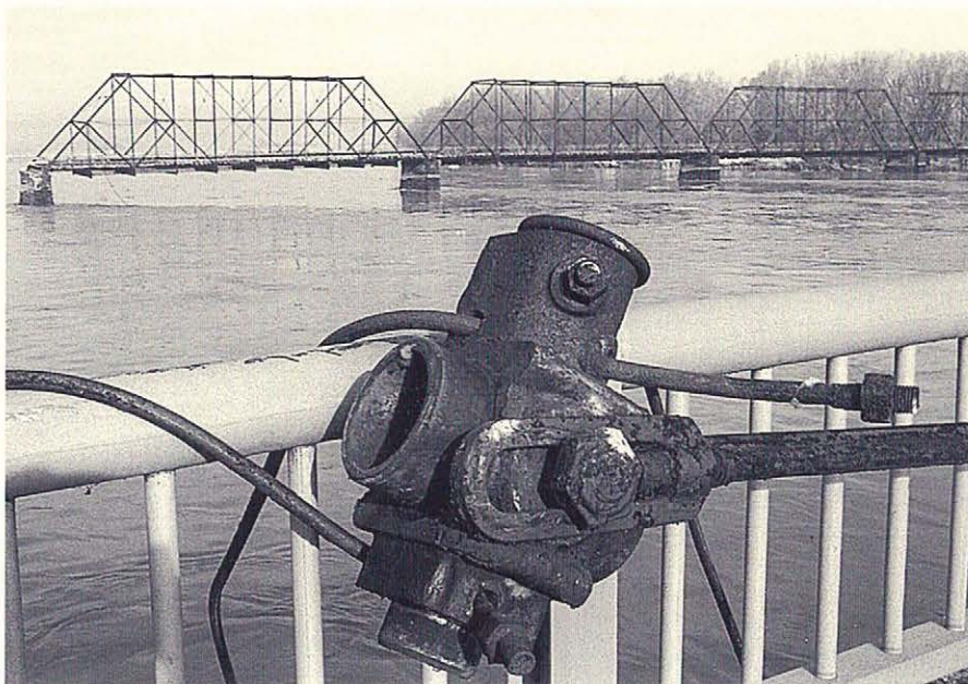
A cast-iron connecting piece of the Walnut St. Bridge is wrapped around the railing of the Market St. Bridge.
