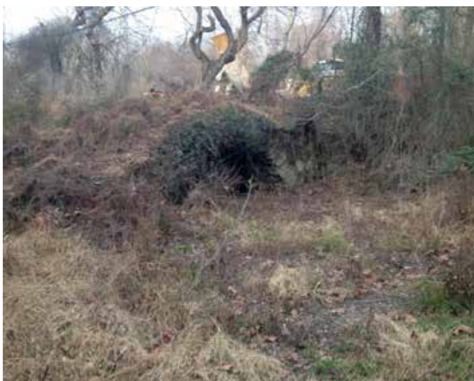
C&D Canal Feeder Bridge (1803-05), vine-covered and largely forgotten in 2016.
