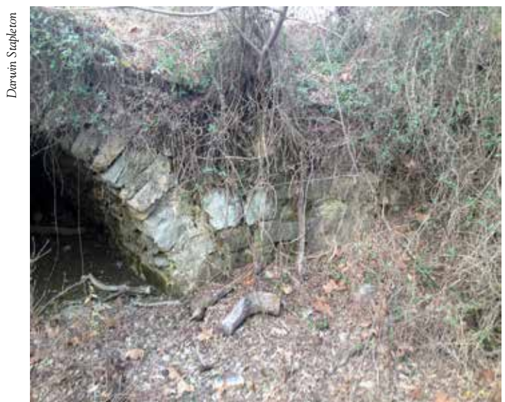
Detail of feeder bridge masonry.
