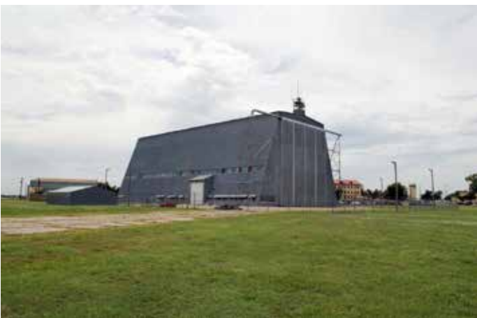
Balloon Hangar at Henry Post Army Airfield.
