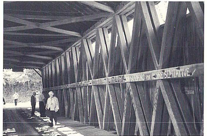
Bennett's Mill Bridge in Greenup County, Kentucky. The unusual three-chord Wheeler truss is visible in the interior view (below). Photos by B.J. McKee (above) and M.F. Wood (below) for Ohio Historic Bridge Assn.
