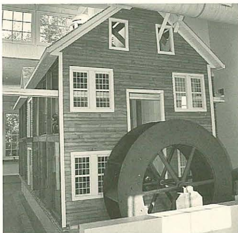
ht: Model end view, wing Whitney's iron erwheel, 14 ft. diam. x 6 ft. le in the original. R.B. rdon photos.
