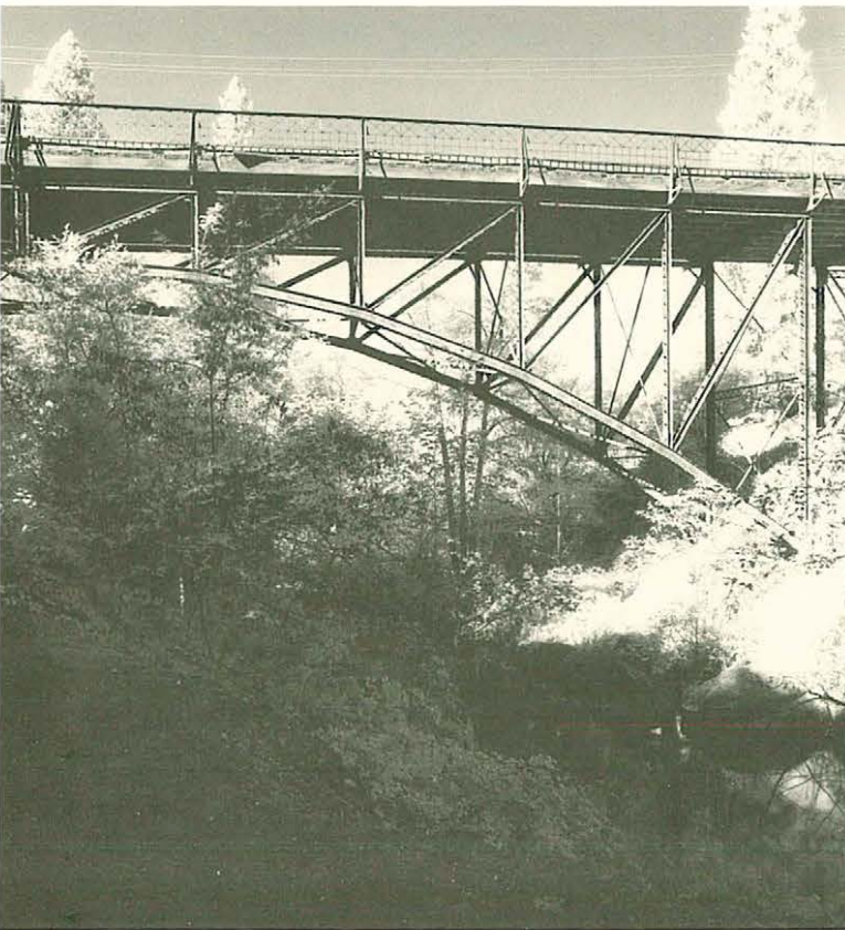
Two views of the historic c1903 Gault Bridge [NR] in Nevada City, Calif., the oldest three-hinged steel-arch truss in the state. The images were recorded on infrared black and white film, rendering the foliage lighter than produced by conventional film. T.L. Peck photo for Foster Engineering, Inc.
