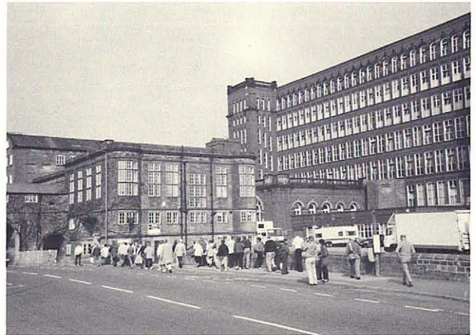
Above: Cotton mills at Belper, birth- & workplace of Samuel Slater: small iron-frame North Mill (1804) & larger steel-frame East Mill (1912). G. Weinstein photo.
