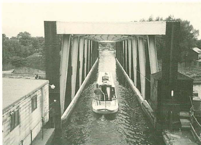
BARTON AQUEDUCT SWING BRIDGE (1893), carrying the Bridgewater Canal over the Manchester Ship Canal, Trafford park, suburban Manchester. The views above show the bridge in its closed position, carrying canal and boat. The views below show it beginning its swing to an open position to allow passage of a vessel below. Span with water weighs 1,450 tons. Black & white images don't do justice to this amazing structure, with its pink diagonals and top bracing, white upper chord, and black lower chord and end posts. Photos by G. Weinstein (above), J. Freeman (below left), & E. Kutsch (below right).
