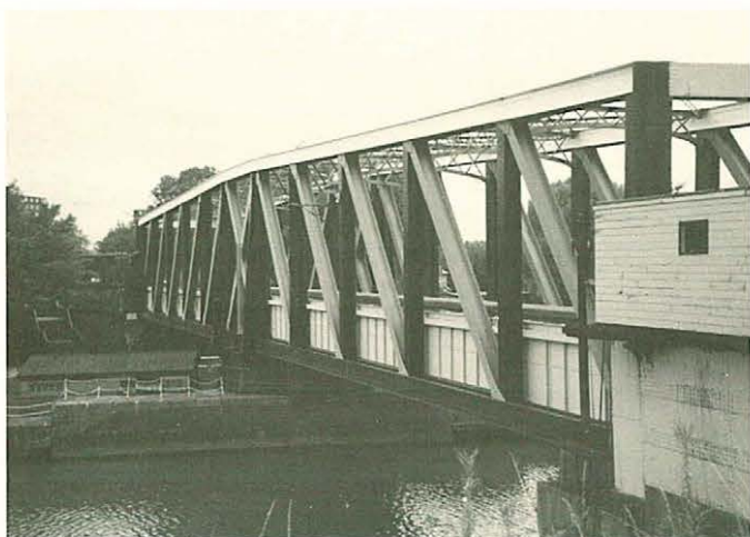
BARTON AQUEDUCT SWING BRIDGE (1893), carrying the Bridgewater Canal over the Manchester Ship Canal, Trafford park, suburban Manchester. The views above show the bridge in its closed position, carrying canal and boat. The views below show it beginning its swing to an open position to allow passage of a vessel below. Span with water weighs 1,450 tons. Black & white images don't do justice to this amazing structure, with its pink diagonals and top bracing, white upper chord, and black lower chord and end posts. Photos by G. Weinstein (above), J. Freeman (below left), & E. Kutsch (below right).
