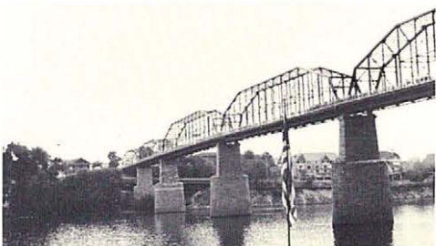
WALNUT ST. BRIDGE, CHATTANOOGA. Left: The 2370-ft., six-span camelback Pratt truss. Right: Crowds celebrate the $4.5-million restoration on May 1, 1993. Photos courtesy J.J. Pullaro.
