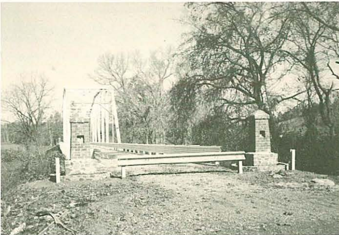
The newly restored camelback truss, located near Sanford, N.C. The gateposts of locally quarried sandstone and locally manufactured brick have recesses for sculpture by an area artist. Ms. Baldrick photo courtesy of W.J. Ellenberger.
