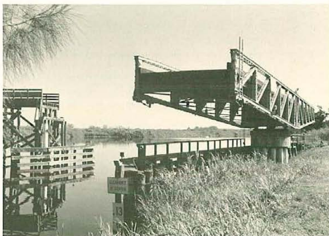
Below: The Torry Island Bridge (1916), the only manually operated Warren pony-truss swing bridge still in use in Florida, was relocated to the Lake Okeechobee Rim Canal at Belle Glade in 1935.
