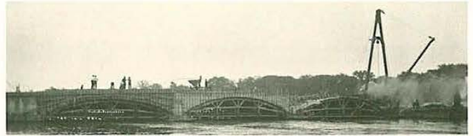
Above: Spandrel-wall forms are erected for the Barrington Bridge, Aug. 30, 1913.
