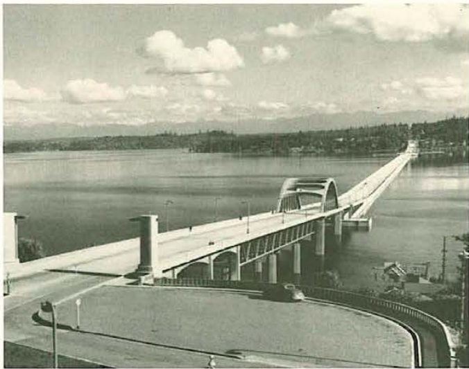
The Floating Bridge included conventional, fixed approach-spans at each end. This view from the Seattle end was taken several months after the official opening in July 1940. Museum of History & Industry, Seattle.
