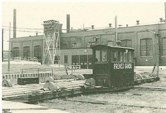
Above: An electrically powered transfer table travelled between Angus Shops' two major buildings.
