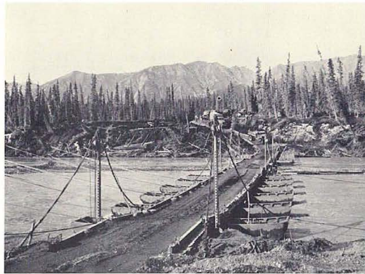
Above: Shore lines anchor this pontoon bridge across the Donjeck River, Yukon, in 1942. Yukon Archives.
