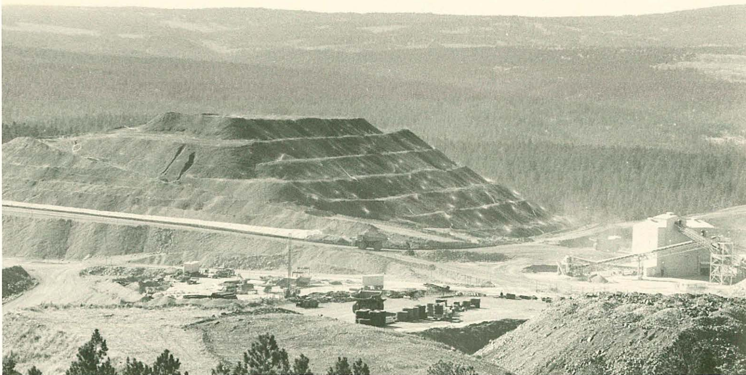
Wharf Resources' heap-leaching process creates an immense pyramid (above) of crushed, previously mined, gold-bearing rock. A solution of 100 ppm of sodium cyanide is passed through the "heap" to leach out the gold. The solution is collected and the gold retrieved. Below is the cyanide neutralization pond. Hamilton & Eisenpress photos.
