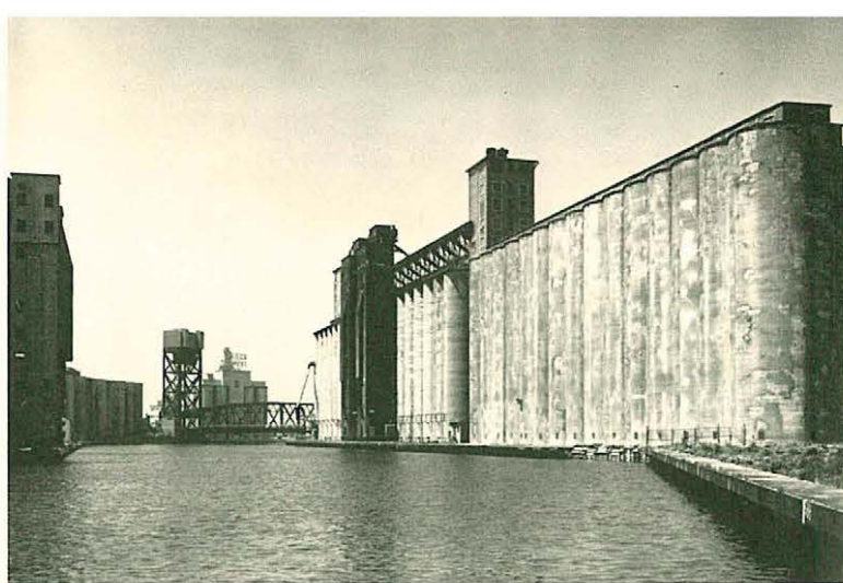
The Standard Elevator (1928, 1941), in the Buffalo River Elevator Dist., is one of four still unloading vessels with mechanized marine legs and scooper gangs. Jet Lowe photo for HAER.
