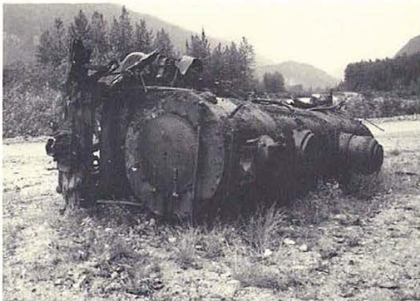
Above: A narrow-gauge WP&YR locomotive (Baldwin, c1900), scrapped in the 1940s and used as rip-rap along the riverbank at Skagway, Alaska. It and another hulk have since been hauled out. P. Malone photo.
