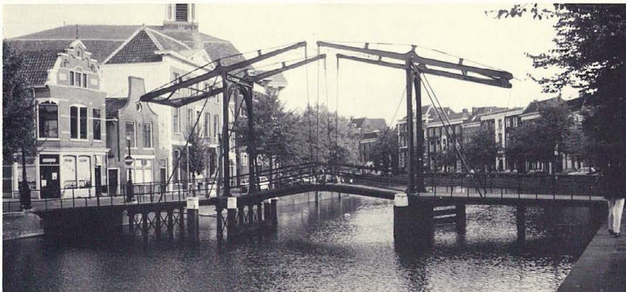
Schiedam: a typical Dutch double-leaf bascule so widely used in the Netherlands to carry roads over canals and rivers, a bridge type essentially unchanged for centuries, whatever the scale or material. This 1873 example is of cast iron. R. Vogel photo.
