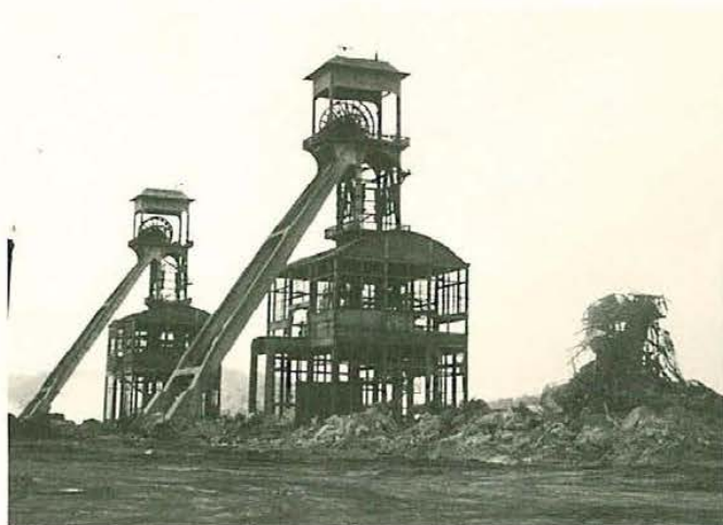
Above: Reinforced-concrete headgear (1920) at the "Limburg-Maas" coal mines of Eisden, province of Limburg, Belgium. Coal-washing plant was reduced to the twisted rubble at right the day we visited. S. Victor photo.
