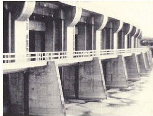
Upstream face of spillway gate structure at Fort Peck Dam. Photo courtesy Jane Morley, ASCE.
