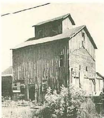
Wood-cribbed elevator (1884), Oconomowoc, Wis., during demolition. Note cribbing on end. Ocono. Enterprise photo.
