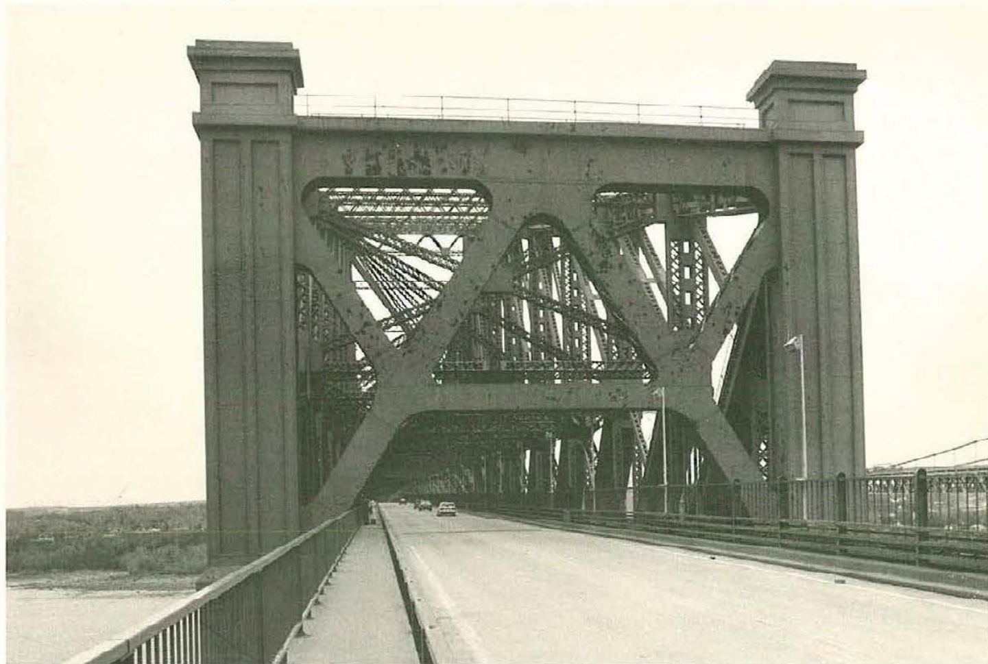
The massive portal of the great Pont de Québec, the Québec Bridge, longest cantilever span in the world (1,800 ft.), and an International Civil Engineering Landmark. Turn page for more photos of this extraordinary structure. R. Frame photo.
