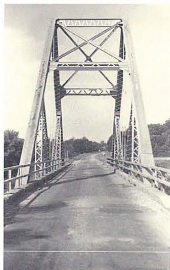
The Missouri Waddell A-truss in its original 1898 site configuration, on a rail spur that was abandoned in 1939 and converted to highway use in 1953. The bridge was dismantled in 1982. The builder's plate is one of two originals, both now lost. Corps of Engineers photos.
