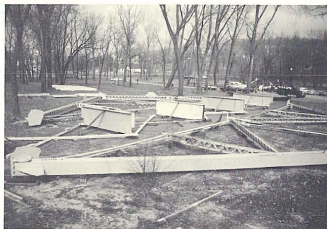
The reassembled trusses and floor-system members, laid out at the new site in late 1987. J. Friedman photo.
