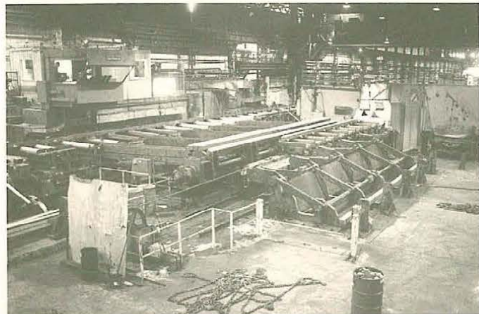
Top, above, & left: Touring the rolling mill at Bethlehem Steel Corp.'s "lower works" in Johnstown, where ingots are worked into blooms and billets. Above right: One of the cavernous abandoned buildings at the Cambria Iron Works. R. Frame photographs.
