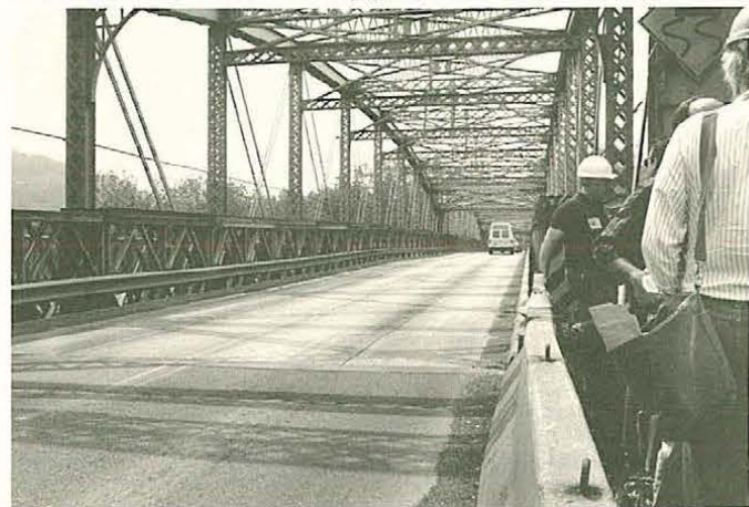
Installed in 1987, a new self-supporting, load-bearing structure made in England carries traffic through the original 1893 trusses of the Bridgeport (Back Channel) Bridge. R. Frame photograph.
