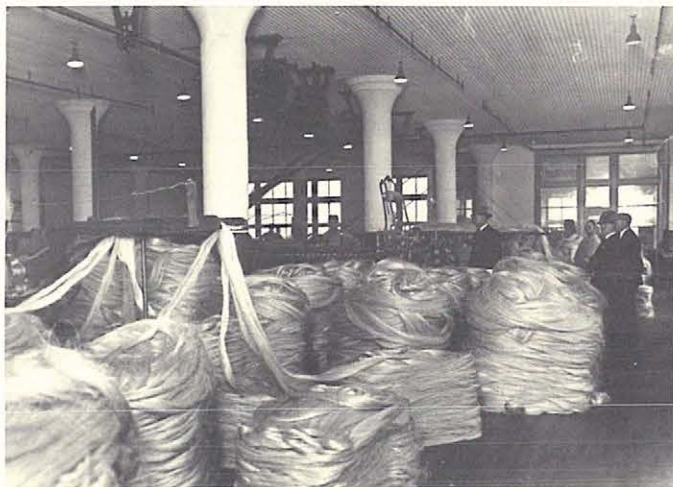
STILLWATER [Minn.] STATE PRISON. Above: Interior of a twine factory building in 1925. Note the concrete flat-slab, mushroom-column construction. Below: The twine warehouse, Bayport, Minn., in 1925. Minnesota Historical Society Collections.
