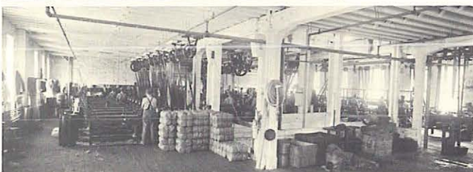
Inside the twine factory at the Stillwater [Minn.] State Prison, c1900, where agricultural twine is being manufactured from hemp. Note the vigilant security officer in the top photo. Minnesota Historical Society Collections.
